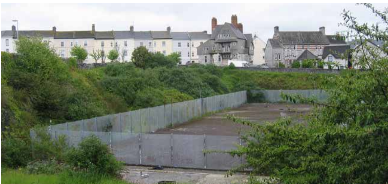
The former sports ground at Stonehouse Arena was a magnet for fly-tipping and antisocial behaviour prior to its redevelopment
